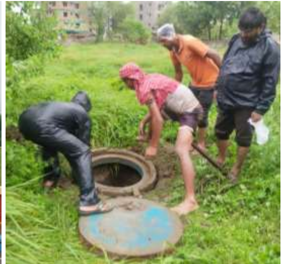
Precautionary Maintenance Work
