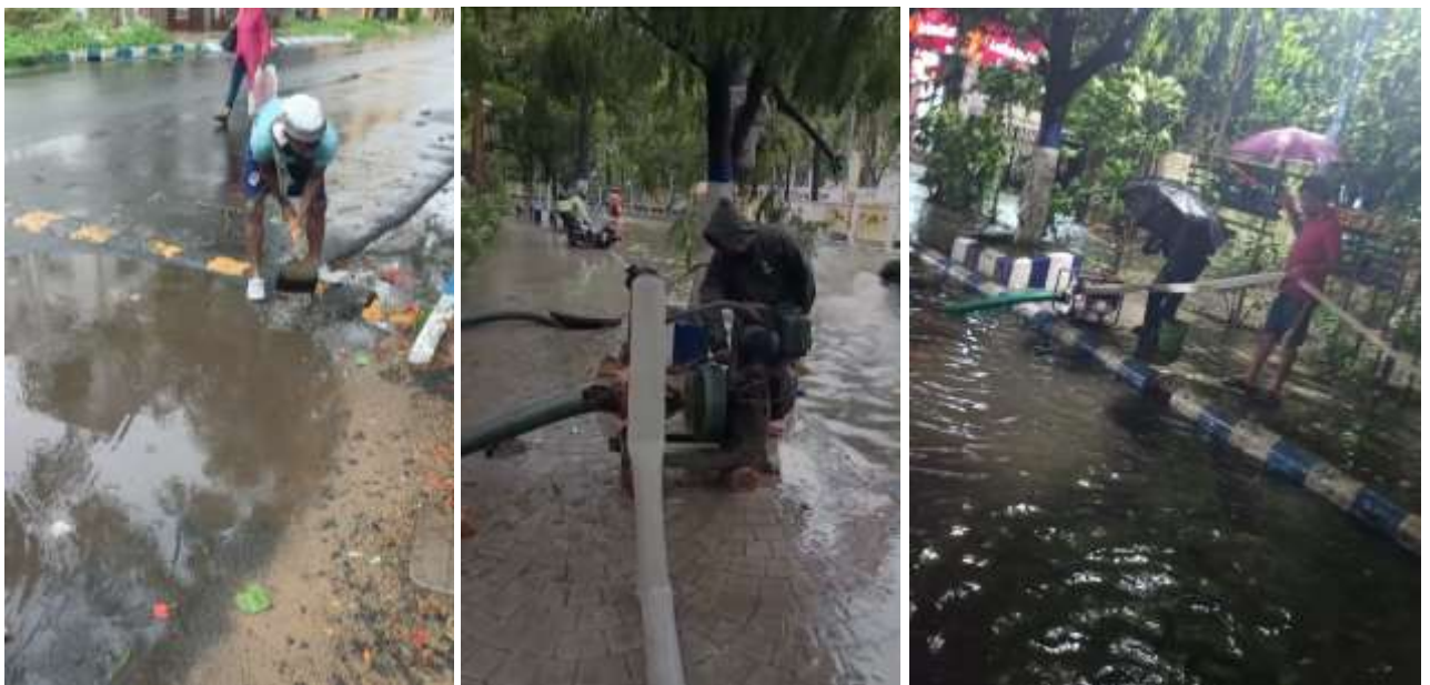
Remediation of Waterlogged Areas by NKDA as an Emergency Service
