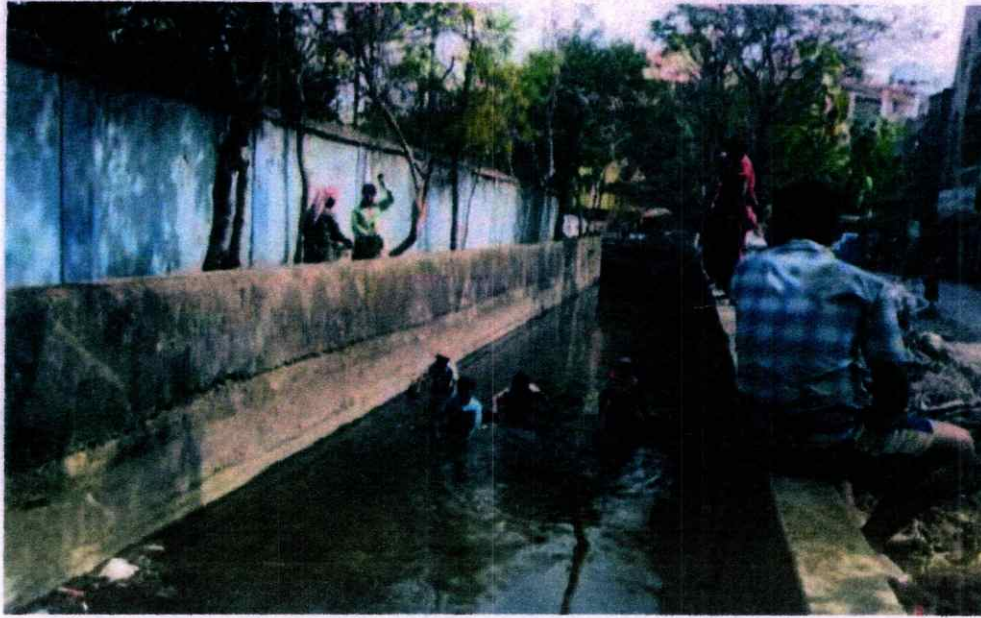
Figure 1 Manual Cleaning of Garbage and Water Hyacinth from Peripheral Canals of New Town
