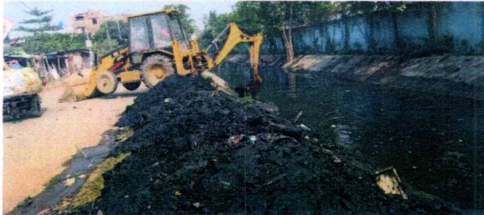
Figure 2 Mechanical Cleaning of Peripheral Canals of New Town
